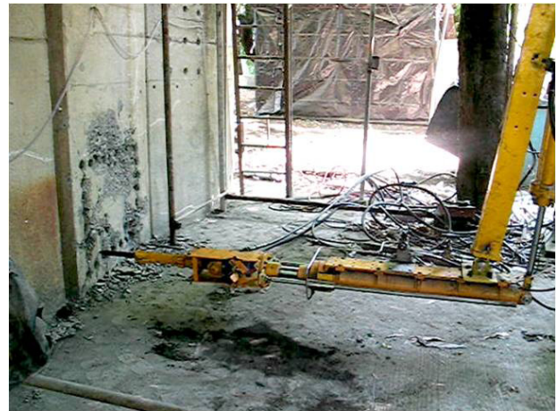
Fig. 2: Breaking/chipping end effector
